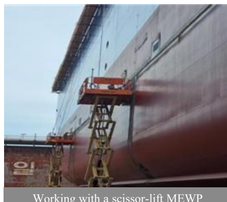
Working with a scissor-lift MEWP
