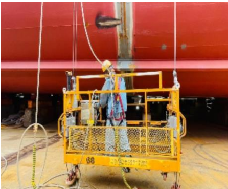
Check for any abnormalities in safety devices and the braking system
