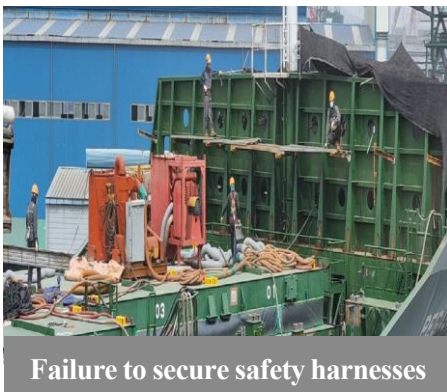
No safety guard rails installed
